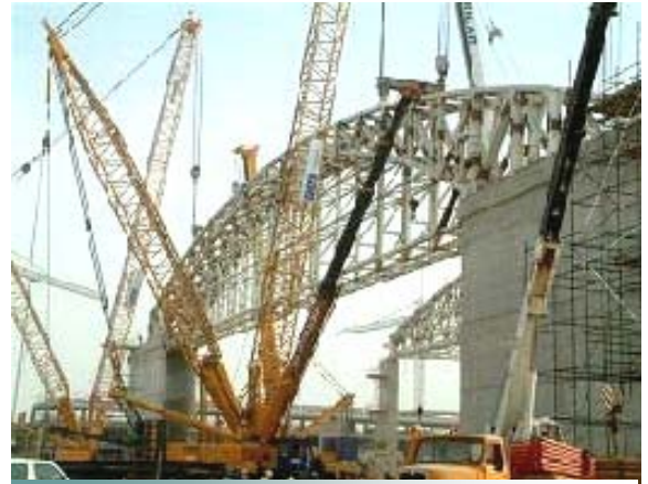
Hangar Facilities for New A380 - Emirates has 40 of the Super-Jumbos on order
