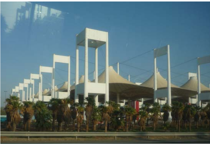
The Distinctive Tented Terminal used by Hajj Pilgrims at KAIA – King Abdulaziz International Airport Jeddah.
